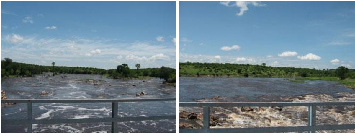
Great Ruaha River | Main Bridge | February 2010
