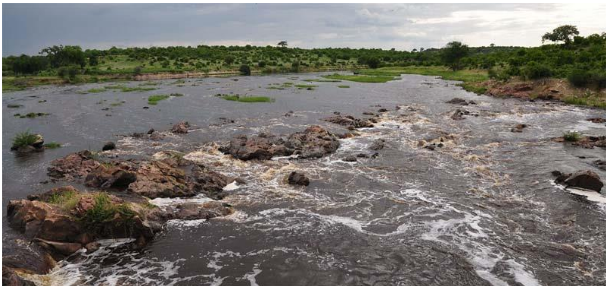
Great Ruaha River | Main Bridge | 6 th February 2012
